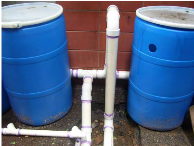
Inflow and outflow pipes connected to the downspout (L). Outflow from each barrel outfitted with a lever to control flow (R).
