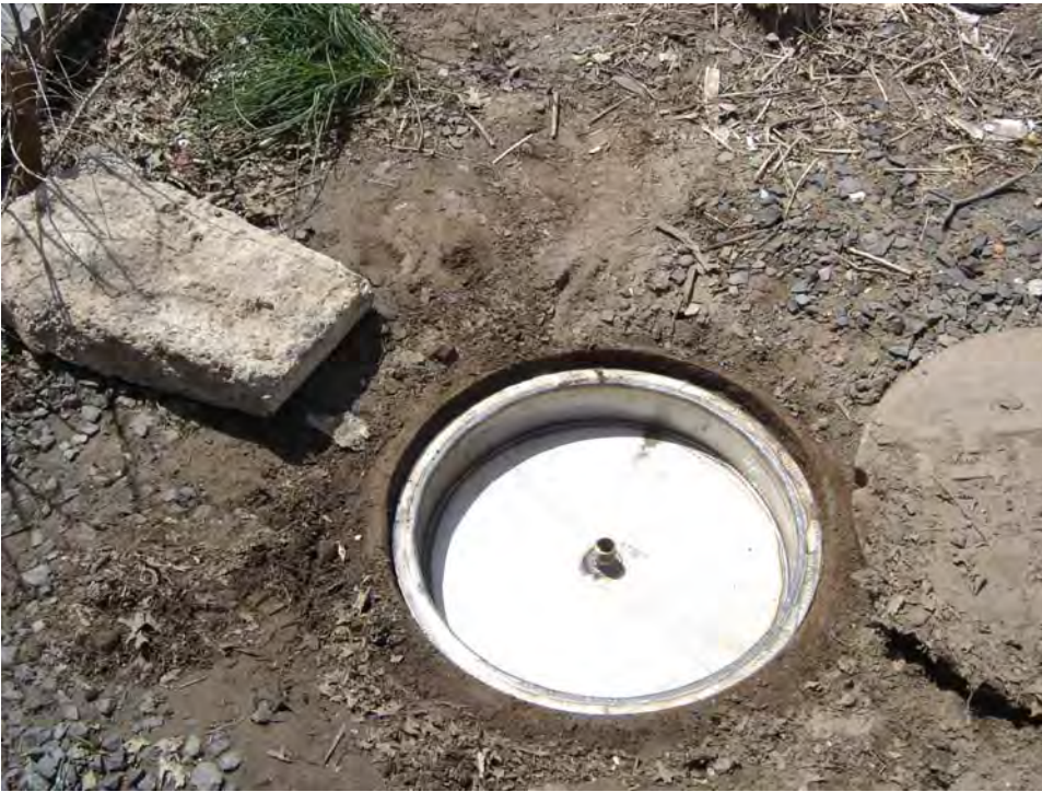
Figure ES-12. Installation of Fabricated Storm Water Insert in Manhole RLD
