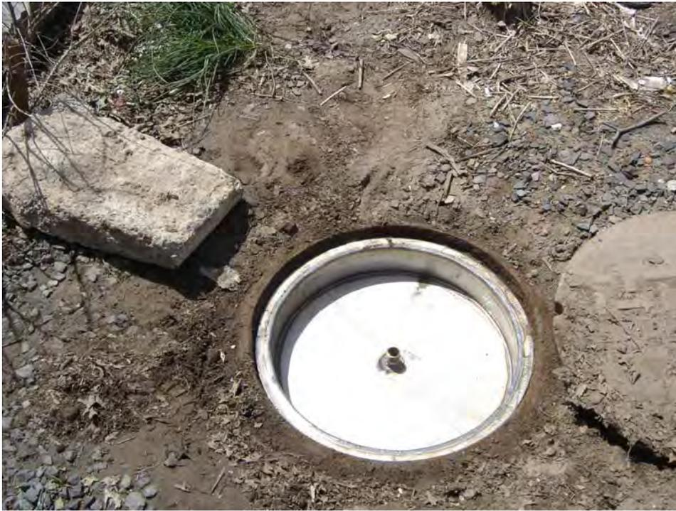
**Figure ES-12. Installation of Fabricated Storm Water Insert in Manhole RLD**
